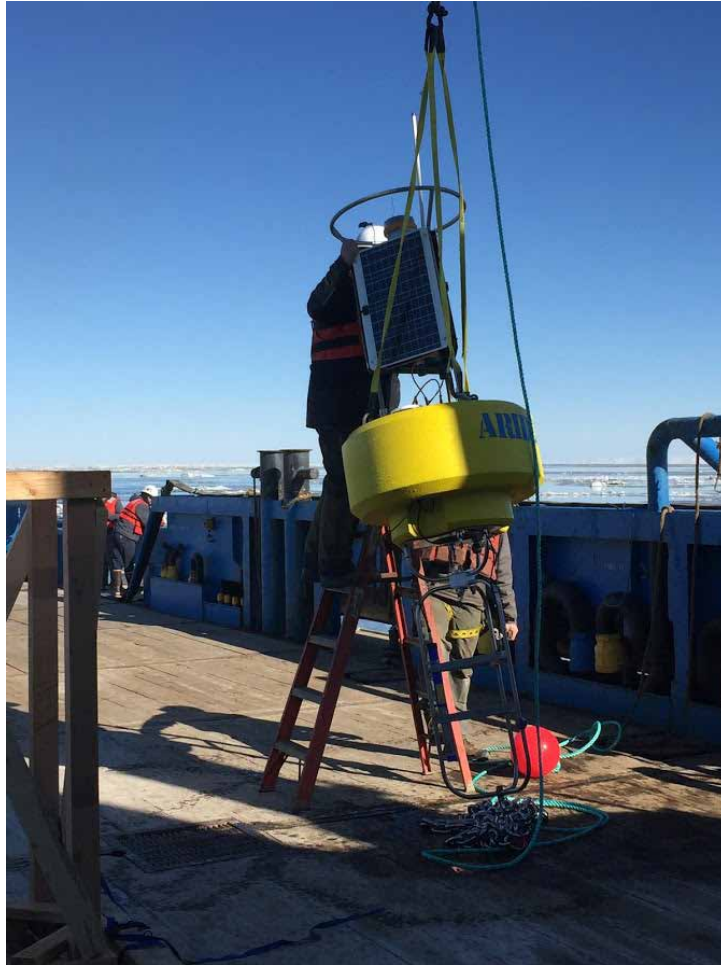
Installation of the buoy at Cook Inlet (Alaska)
