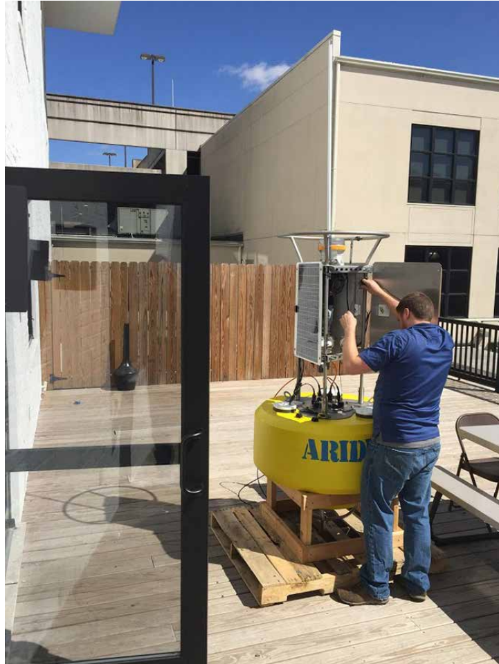
Mounting of the buoy at Aridea's headquarters in West Virginia
