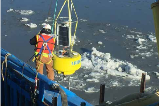
Technicians installing Aridea's buoy in the water
