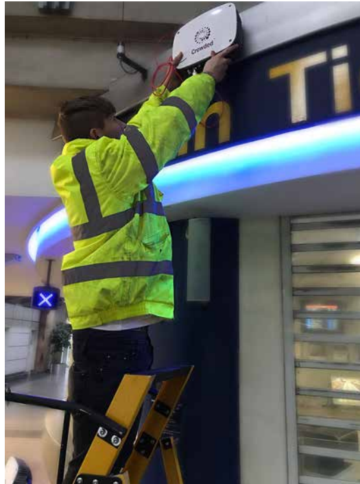
Installation of the Meshlium Scanner - Crowded™ Platform
